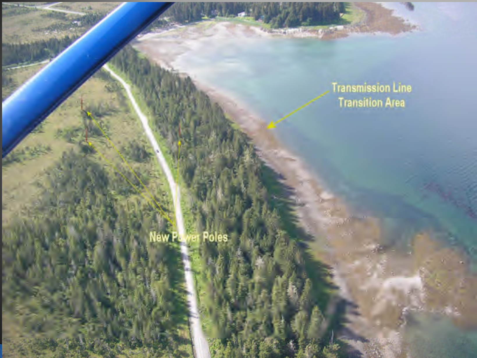
▶ Submarine Cable Landing Near Petersburg
